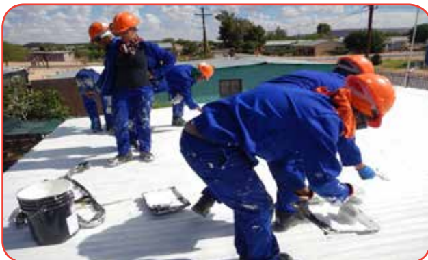
Figure 21: !Kheis Community members using Cool Roof paint for thermal comfort
